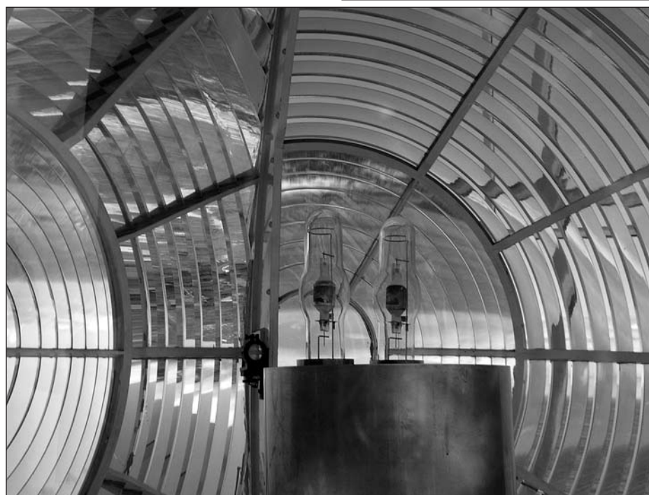
The First Order Lens at Slangkop in South Africa. Photo by the author.
